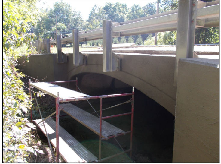
Nimisila Road Bridge Concrete Repair
