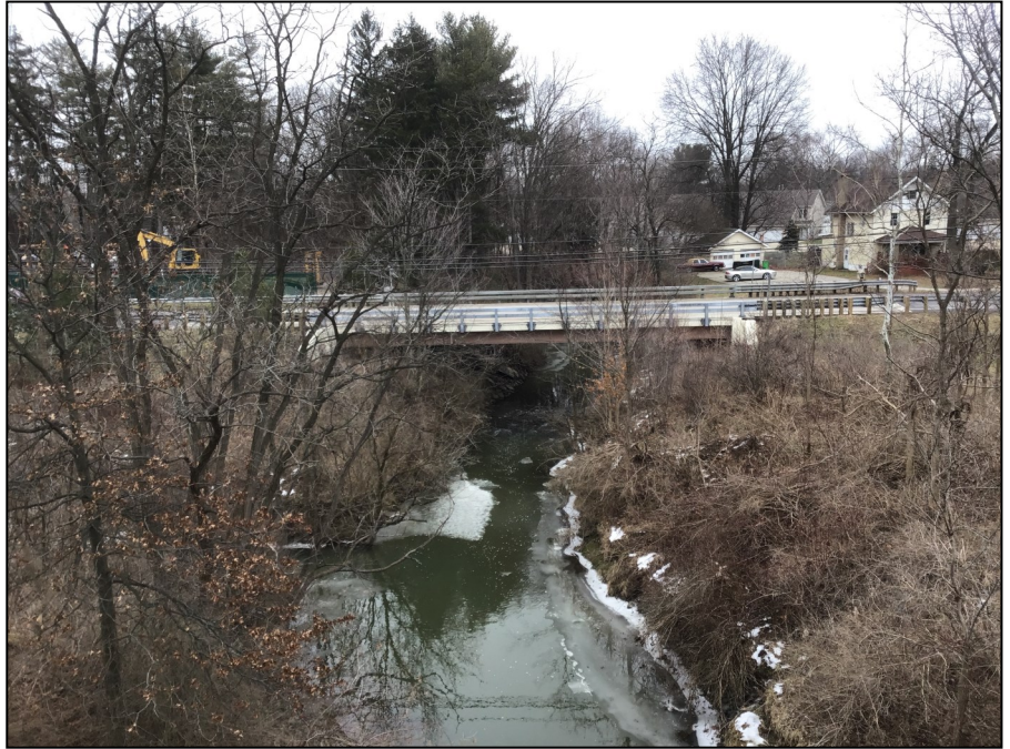
Highland Road Bridge Inspection Photo
