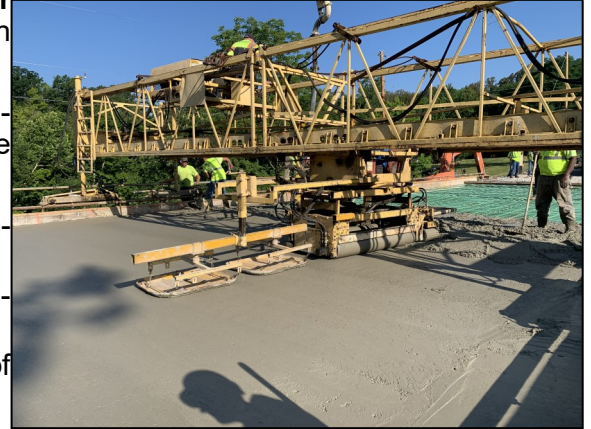
Brandywine Road Bridge over Brandywine Creek— Deck Pour
