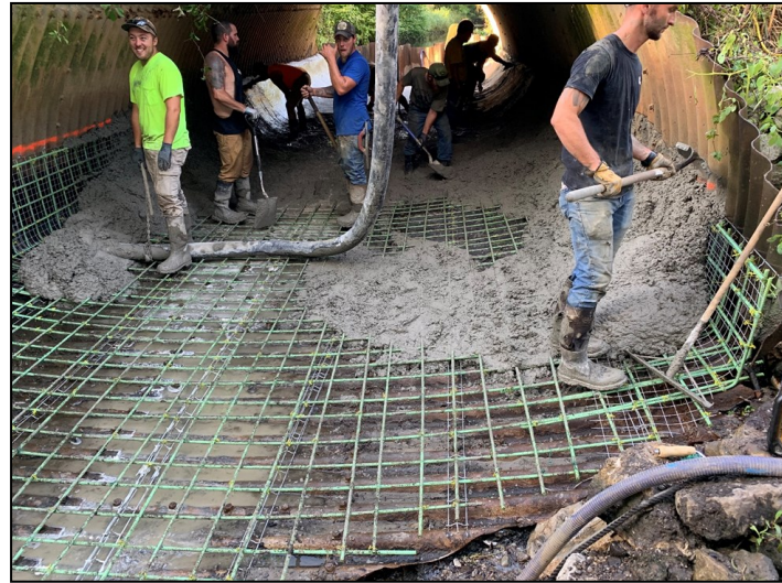
Knox Blvd Concrete Field Paving
