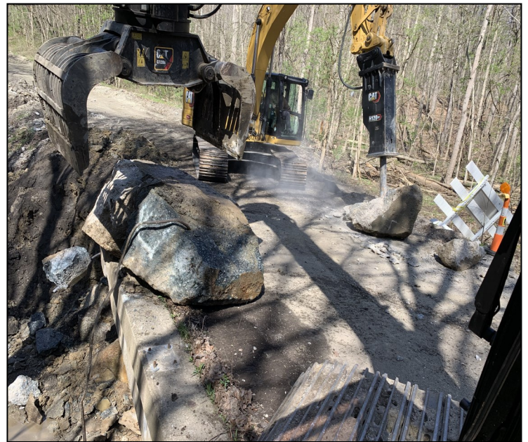
Everett Road Bridge Removal
