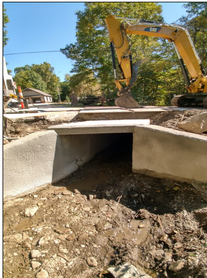
Revere Road Culvert Repair
