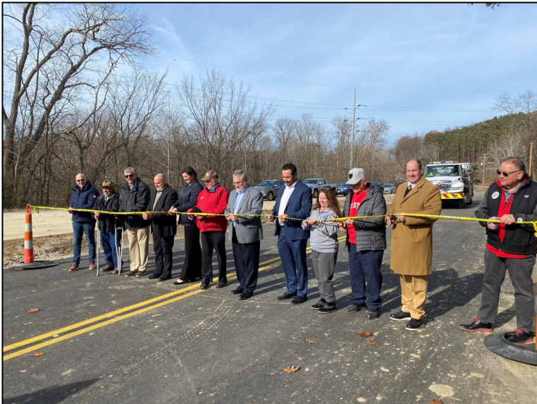
Engineer Brubaker, County, and Village officials at the ribbon cutting ceremony for Akron-Peninsula Road in Peninsula
