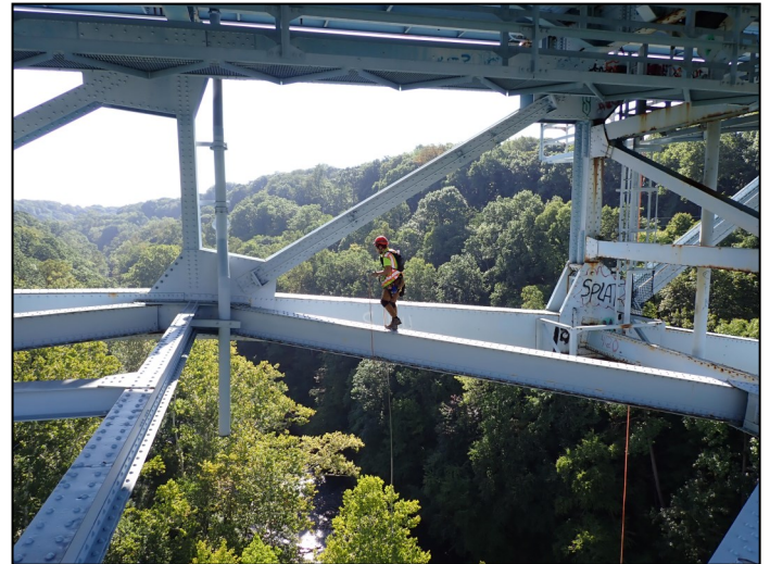
High Level Bridge Inspection
