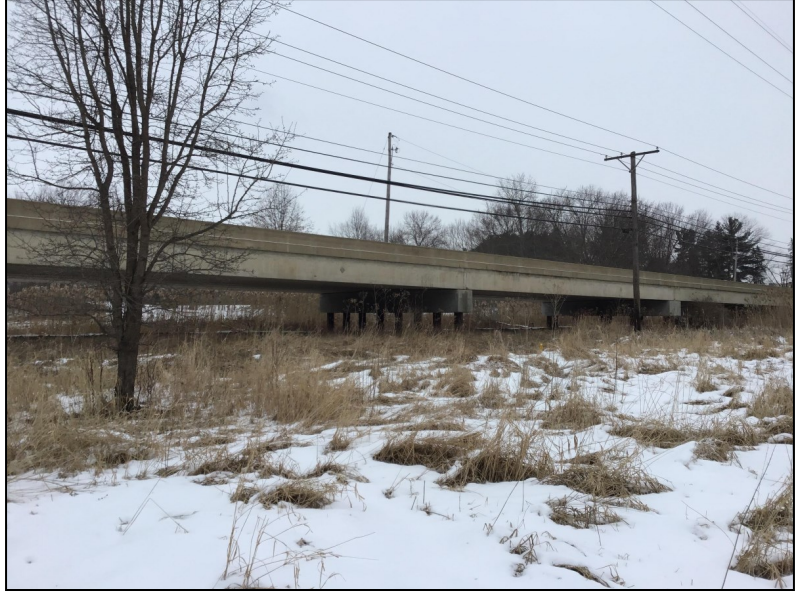
Steels Corners Road Bridge
