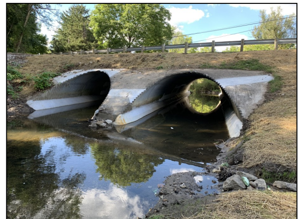
Skelton Road Culvert Concrete Field Paving
