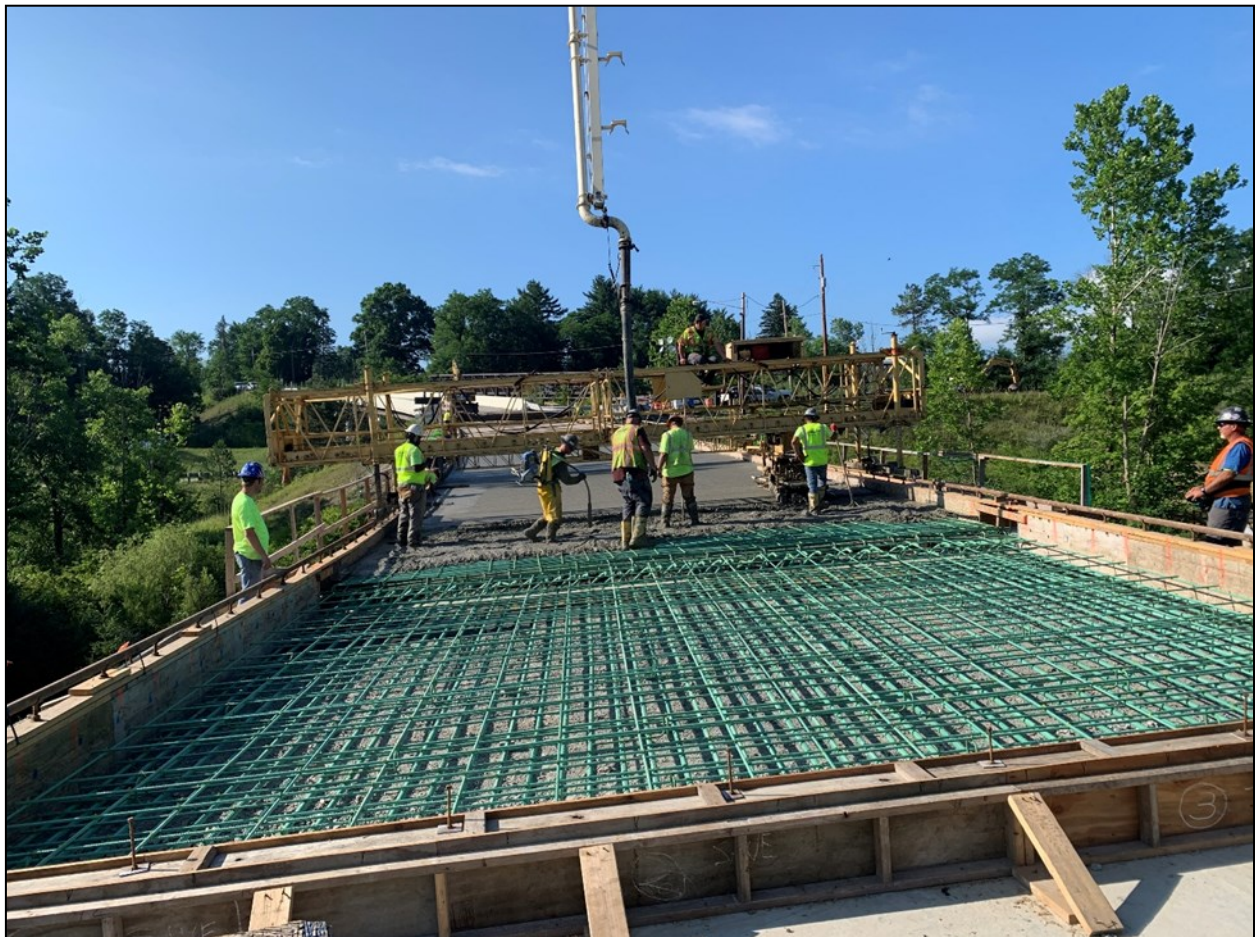
Brandywine Road Bridge over Brandywine Creek
