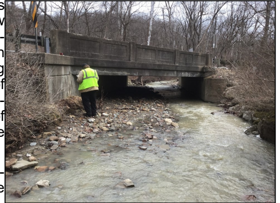
Annual Inspection—Wheatley Road Bridge over Riding Run
