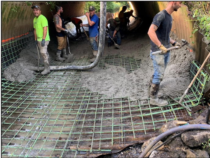
Knox Blvd Concrete Field Paving
