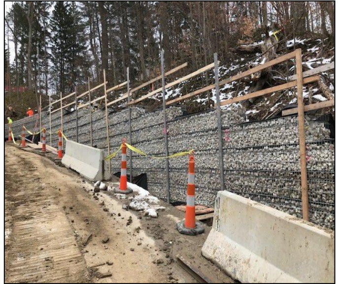
West Bath Road Landslide Repair—Retaining Wall
