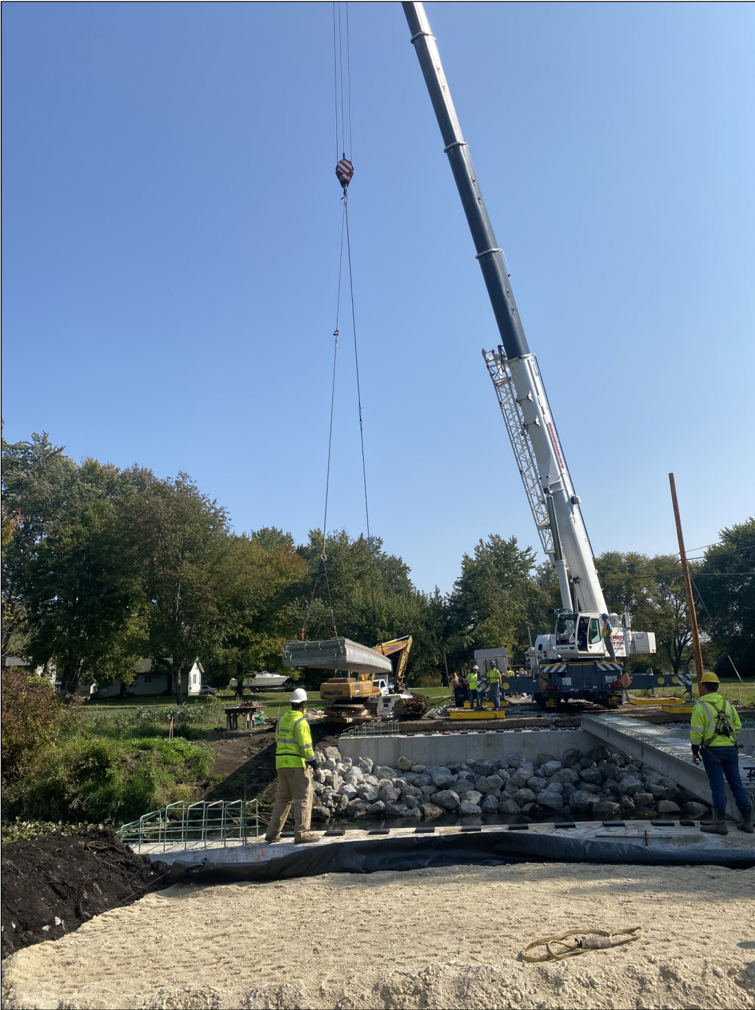
Wright Road Bridge Beam Setting
