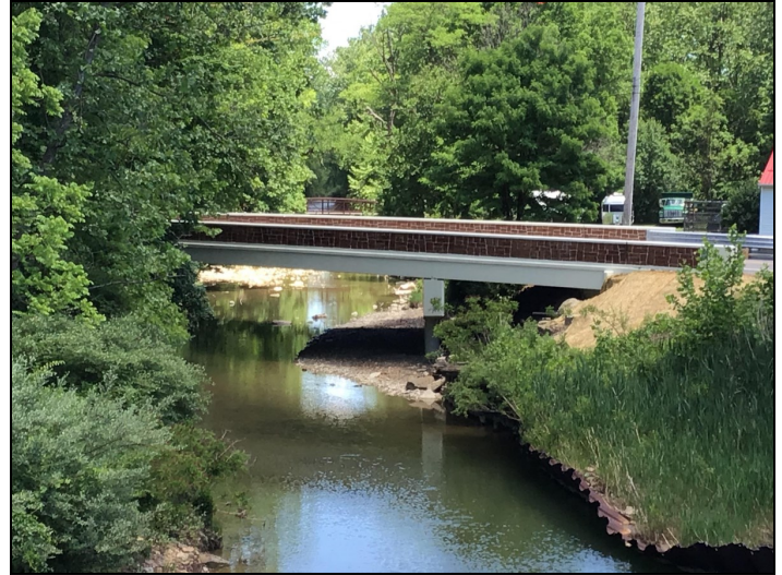
Riverview Road over Furnace Run
