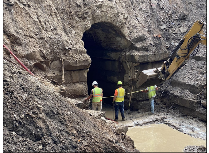
Riverview Road over Slipper Run Emergency Bridge Replacement
