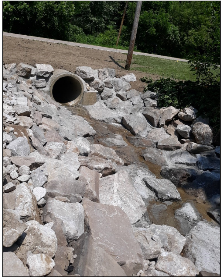
Yellow Creek Road Erosion Repair Project
