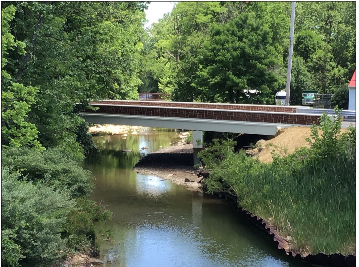
Riverview Road over Furnace Run
