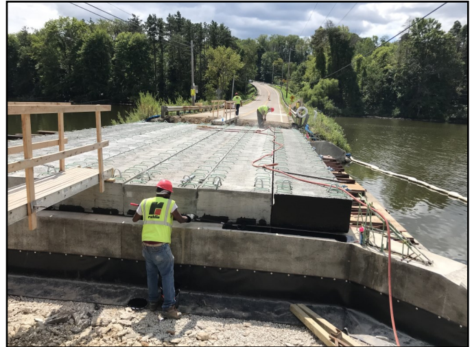
Cleveland-Massillon Road over Wolf Creek Emergency Bridge Repair
