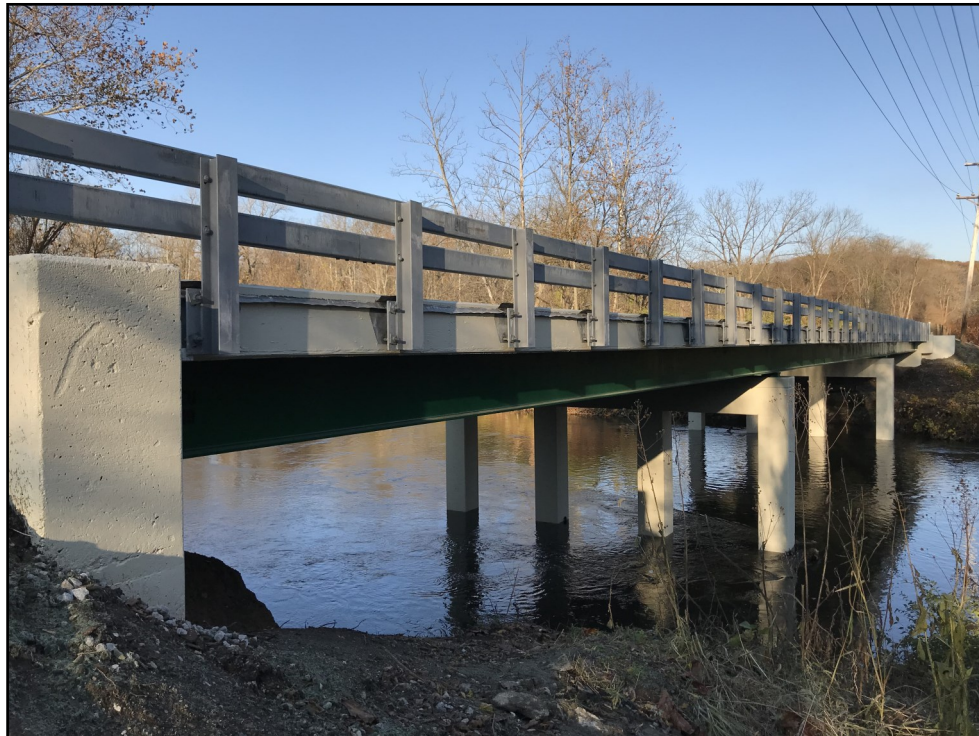
W. Bath Road Bridge Rehabilitation Project
