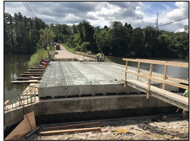
Cleveland-Massillon Road over Wolf Creek Emergency Bridge Repair Project
