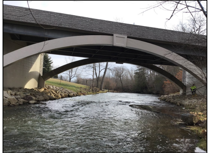
Ravenna Road Bridge over Tinker's Creek—2019 Bridge Inspection
