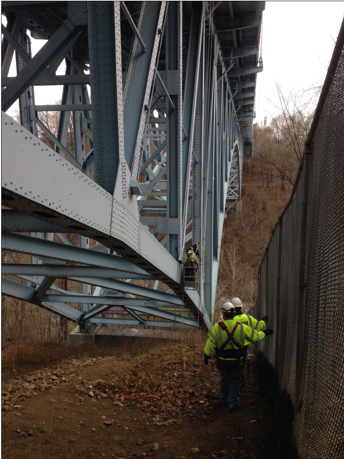
High Level Bridge Inspection
